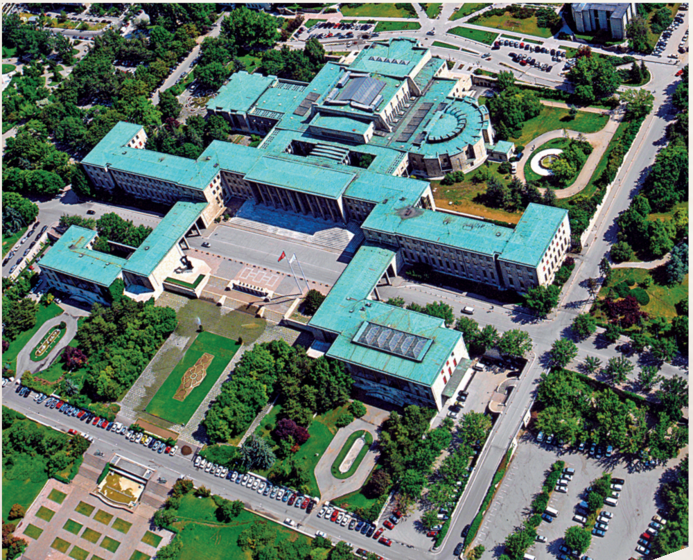
Bird's-eye view of the building of the GNAT
