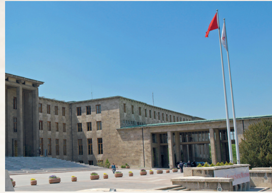
The bridge connecting the building of the GNAT to the Ceremony Hall
