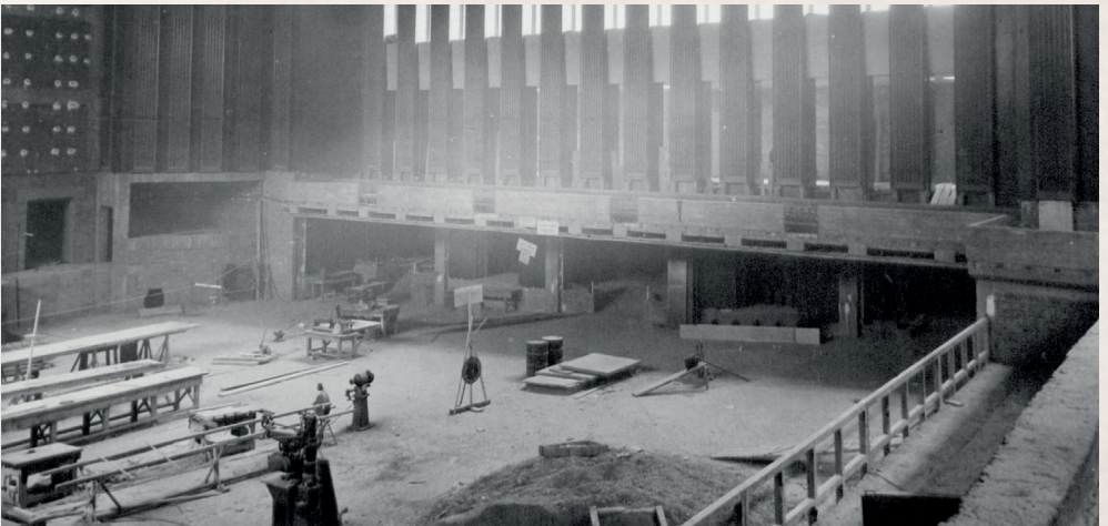
Construction of the Plenary Hall of the GNAT
