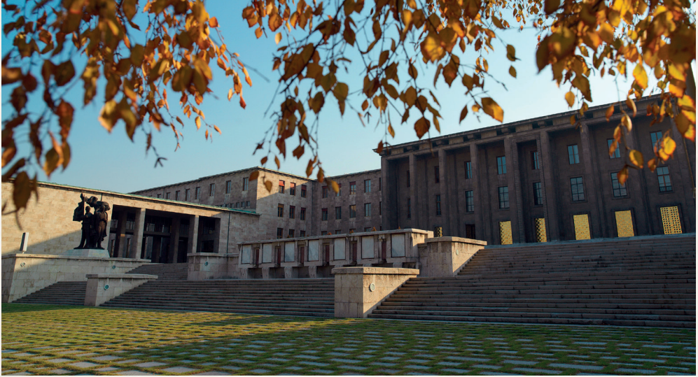
The building of the GNAT
