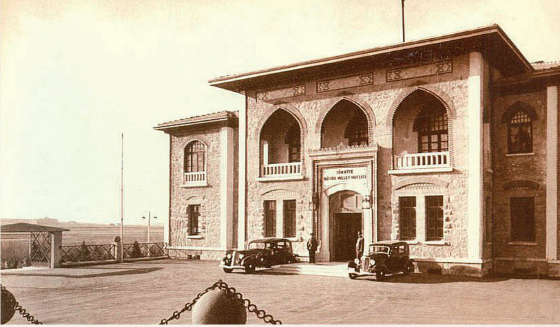
The second building of GNAT
