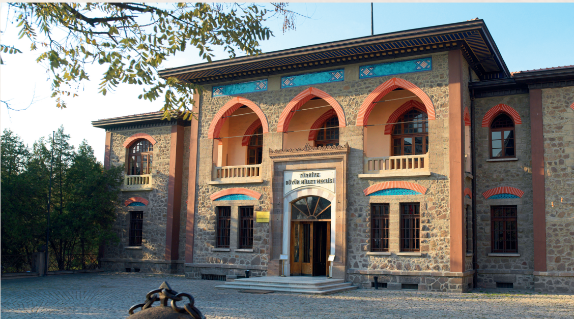
The second building of GNAT (Republic Museum)
